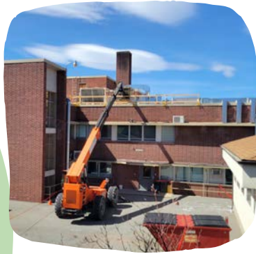
Telehandler helping with demo work on St. Martins Bldg roof
