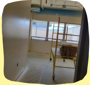
2nd floor St Martins Bldg Office Space
